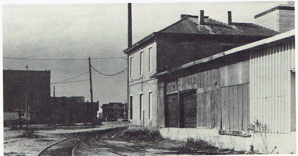
Above, the west elevation of the Katy station. Originally a residence, the building is now half vacant. The south side of the structure, facing the yard, is seen below. The freight shed area is to the right of the station.
